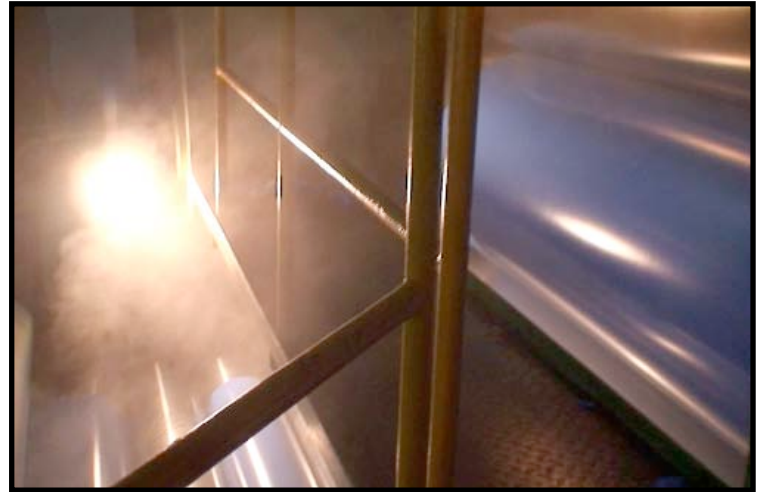
Excess heat emitted by calender machine
